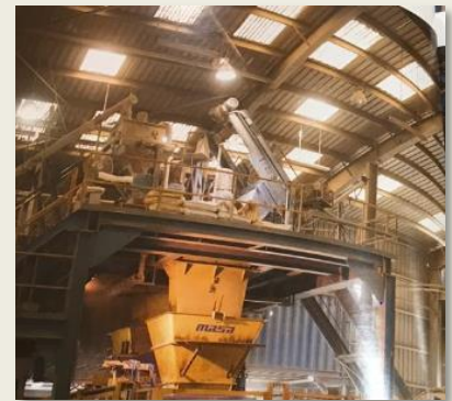
Concrete product factory, Bangalore
