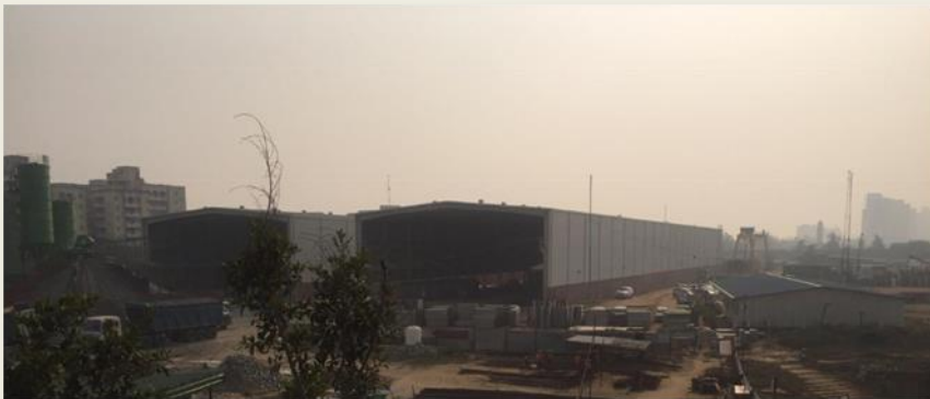
Pre-cast factory at Godrej Golf Links project site
