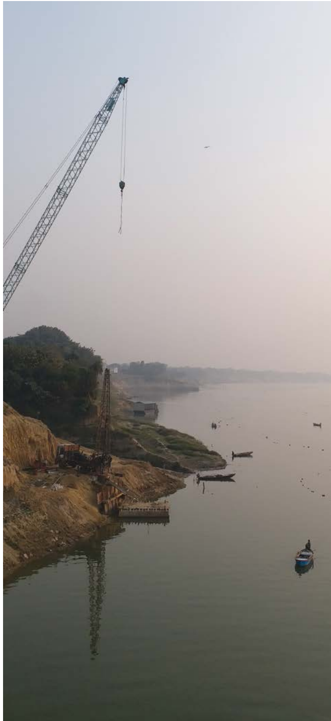
Inland water terminal work on Ganga River at Varanasi
