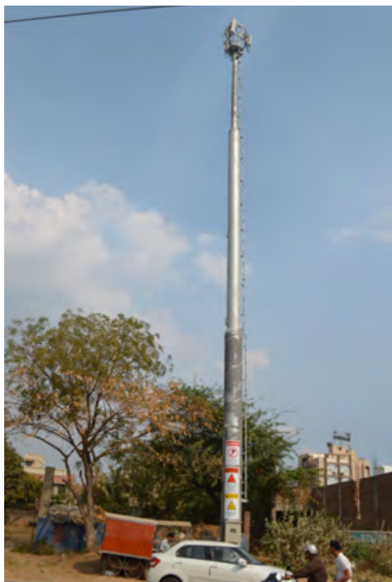
Ground based tower illustration... and live 4G GBM site supporting the service
