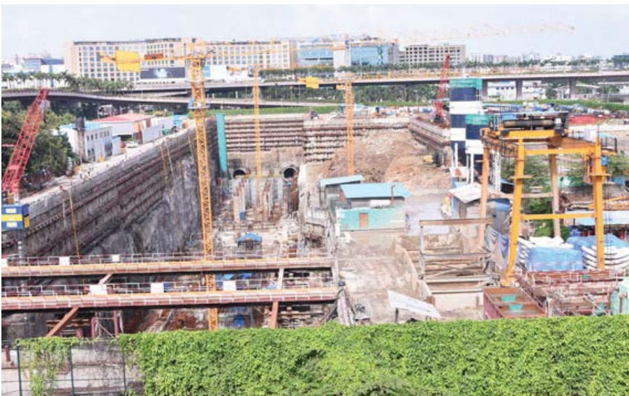
Progress on Mumbai Metro Line 3 - International Airport Site
