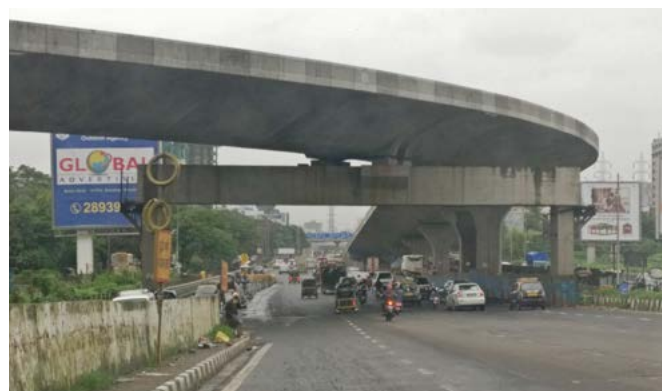
BKC Sion flyover under construction
