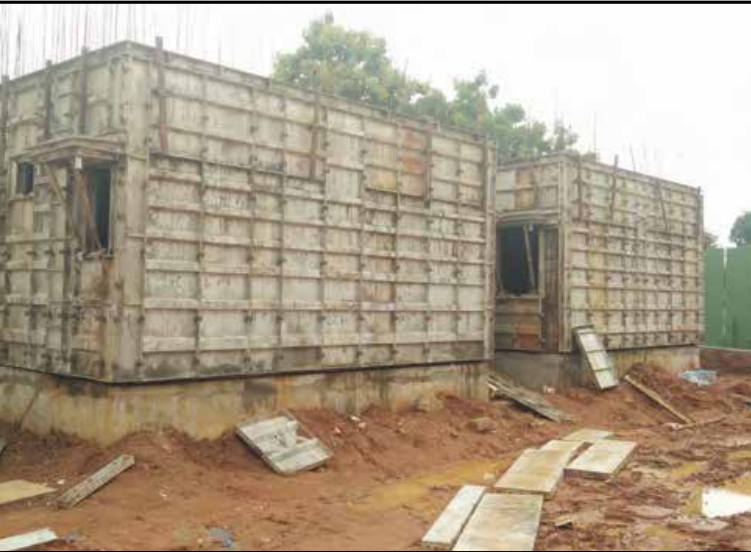
Structure erected from aluminium formworks
