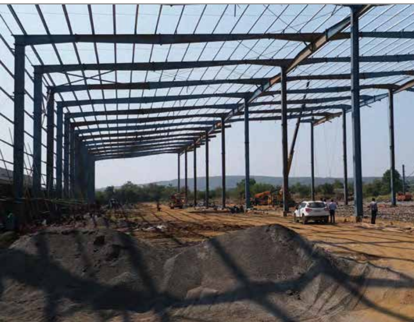
Construction of warehouses with PEB structures
