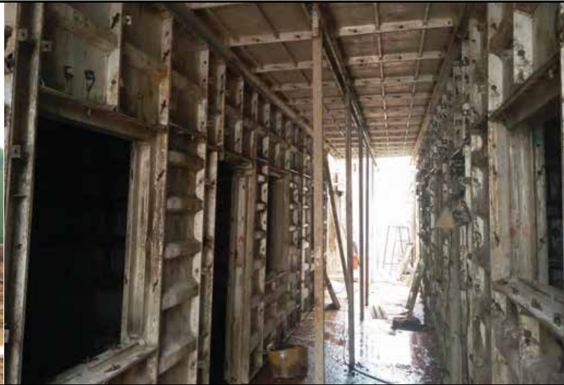
Aluminium formworks used in MIVAN technology
