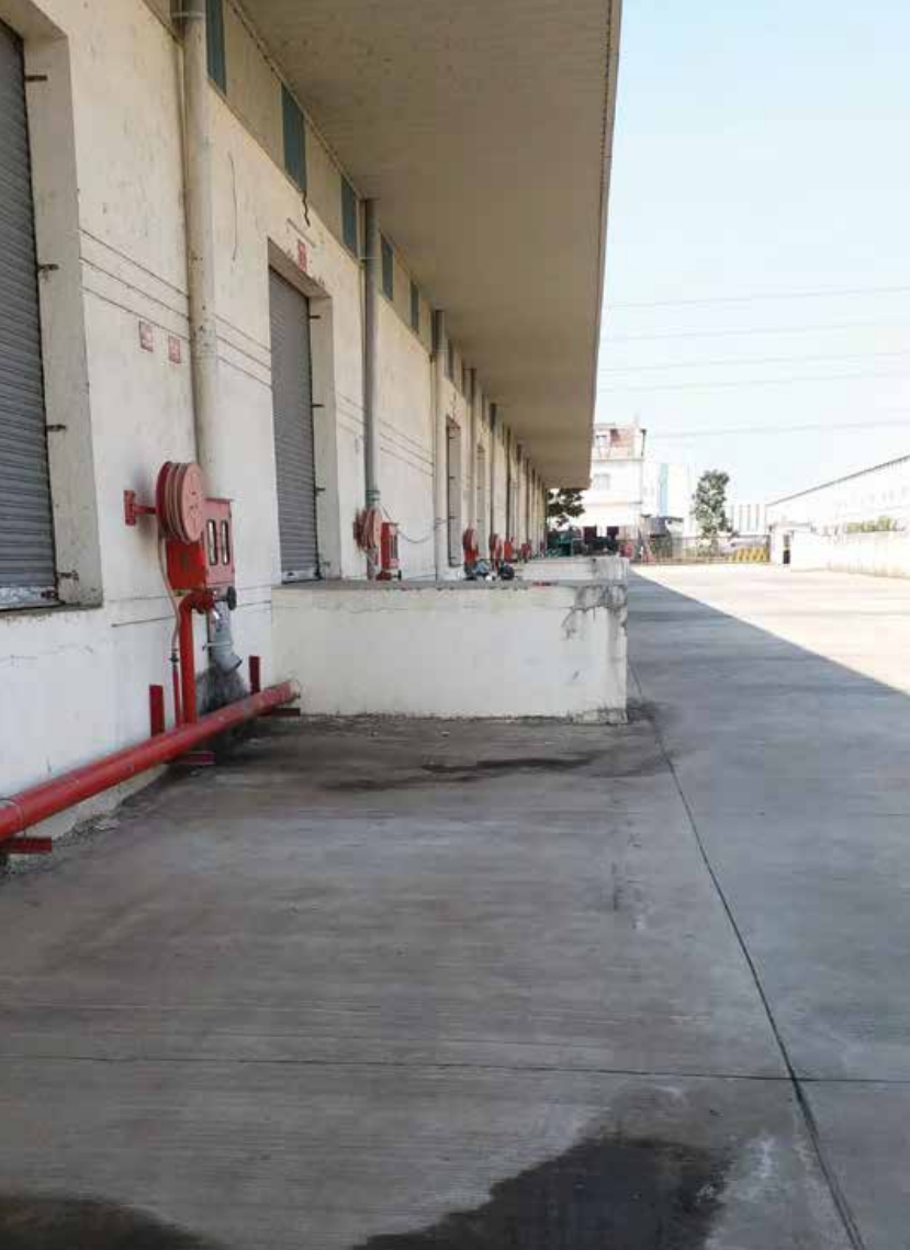
Wider approach road for 40ft containers
