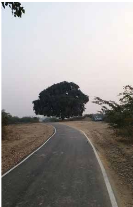
the temporary approach road developed for inauguration
