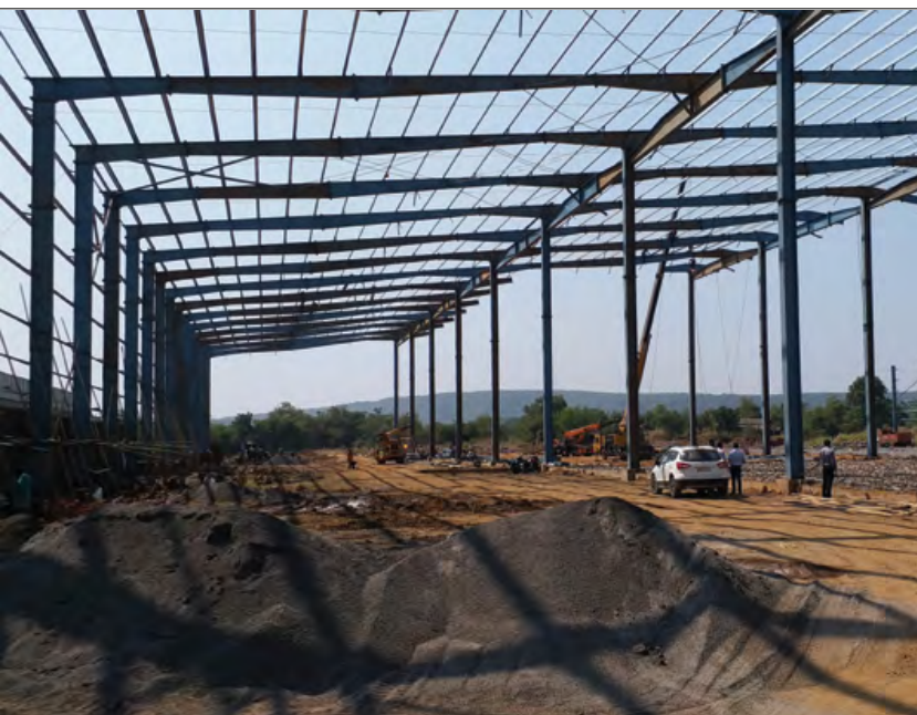
Construction of warehouses with PEB structures
