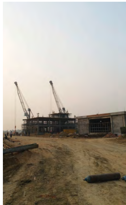
Phase-1 construction - likely to be complete by March 2019
