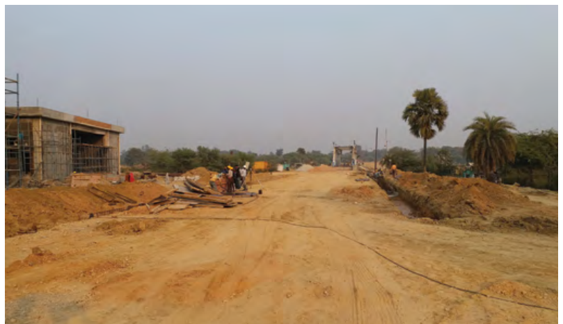
Road construction to the terminal will be complete in 1-2 months
