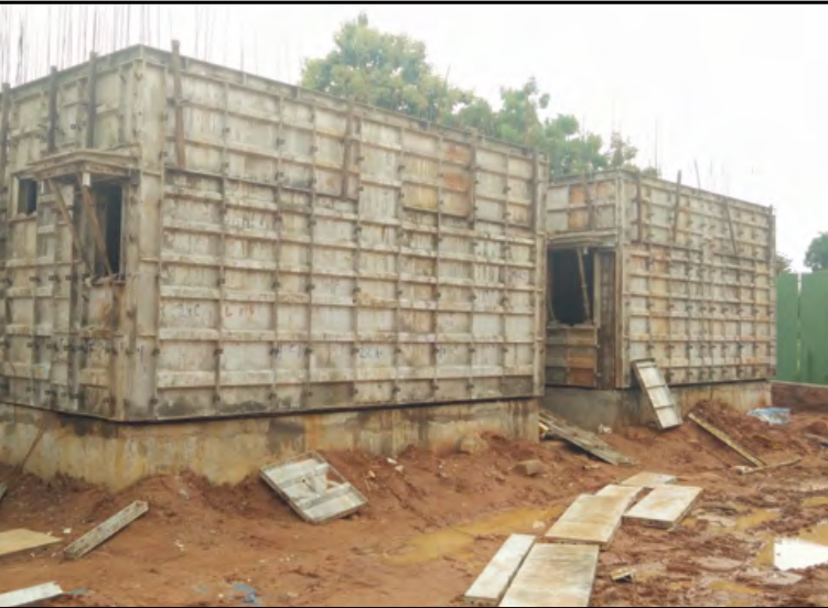
Structure erected from aluminium formworks
