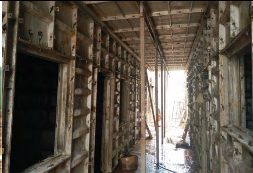
Aluminium formworks used in MIVAN technology
