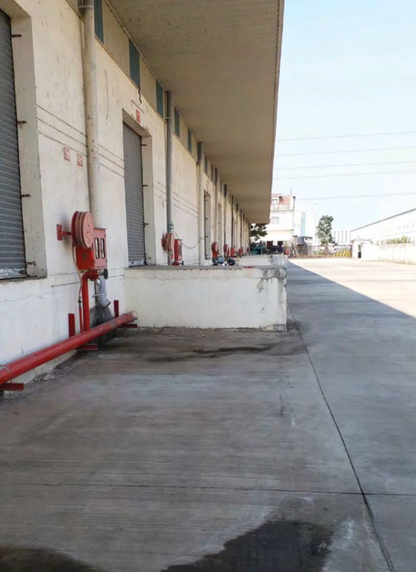
Wider approach road for 40ft containers
