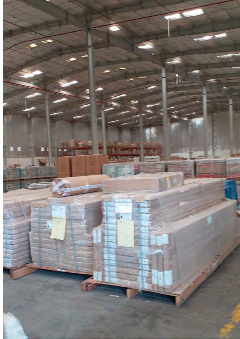
New 'A-grade' warehouses - with natural light, firefighting, drainage systems
