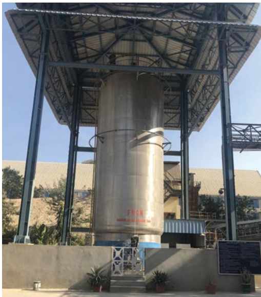
SNCR unit set up to comply with NOx norms. The notice details precautions around the sensitive SNCR site.
