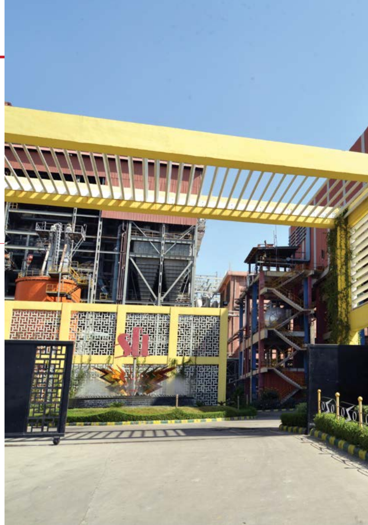
Shree Cement's Mega Power unit at Ras.
