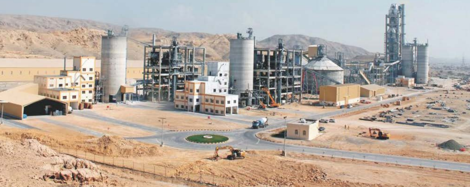
JK Cement's UAE production facility with two parallel lines post clinkerisation.
