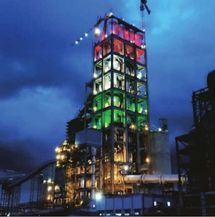
Pre-heater of Shree Cement's South India plant decorated in the shades of The Indian Flag.
