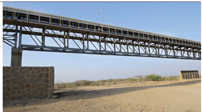
Conveyor belt laid from the mines to the plant as described by the Sanghi brothers to answer a question on incremental cost saving potential for first unit.
